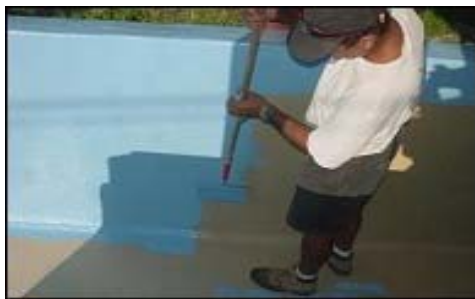
FIGURE 5: ROLLER APPLICATION
